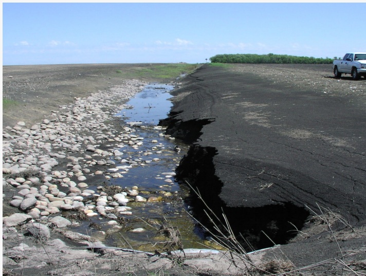
Sedimentation in Kittson County Ditch 26
