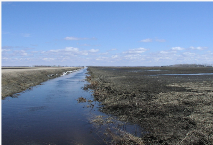
Grass Filter Strip Needed Along a Perennial Flowing Ditch
